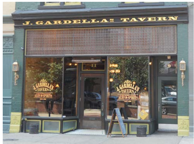
Example of a Historic Storefront
