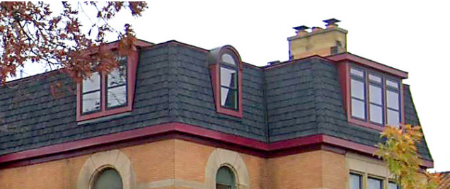
Mansard style roof ▼
