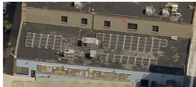
An approved Roof Mounted Solar installation located on flat roof with parapet
