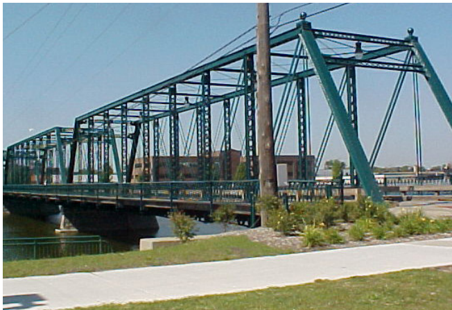
6th Street Bridge, built in 1886 Longest, oldest remaining metal bridge in Michigan
