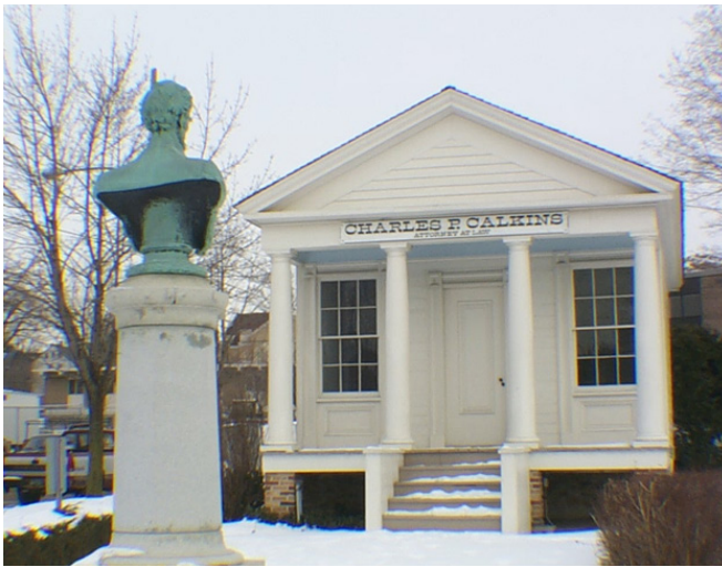
235 State St. SE, built in 1836 The Calkins Law Office is considered to be the oldest remaining frame structure in Grand Rapids
