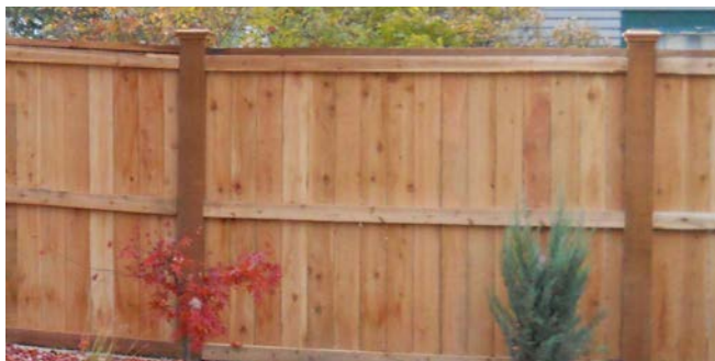
Example of a Wood, Privacy Fence
